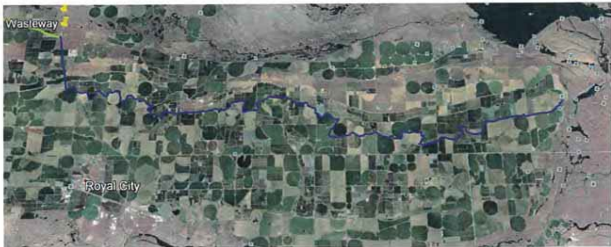
Figure 1 - Quincy Columbia Basin Irrigation District's Lower West Canal
